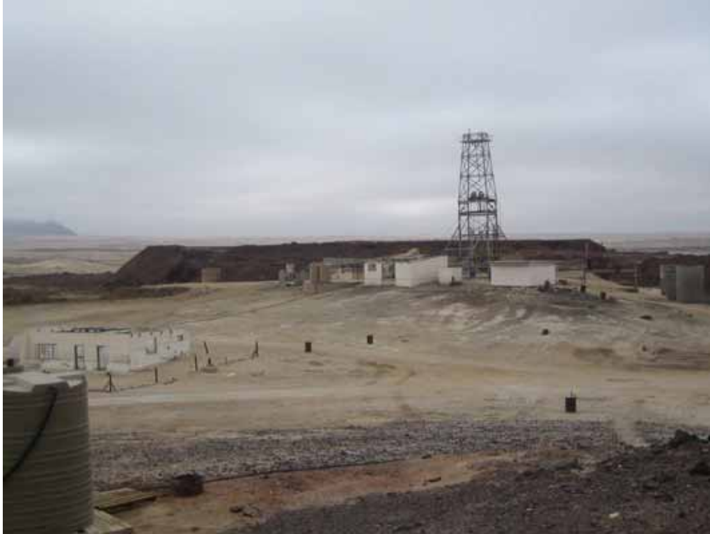
Figure 3-23 Namib Lead Mine Headgear and Tailings Dump
